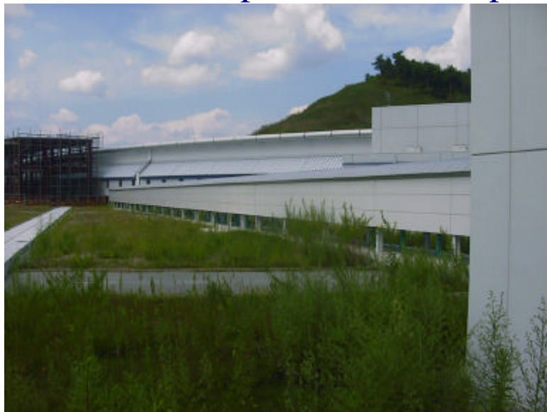
100-meter-long transport channel covered by the arcade in the open (seen from the Biomedical imaging center to the Storage ring building)
